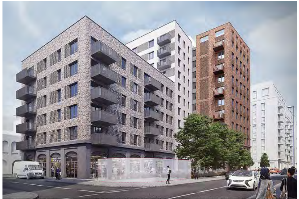
View along Avon Street looking up Providence Place and towards the new piazza space. Existing sub-station is shown in the background.
